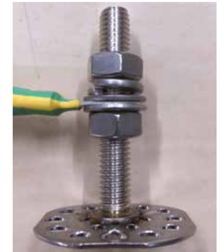
Earth connection point
